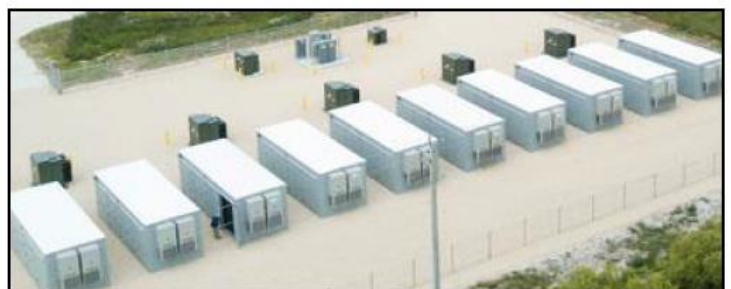
Figure 2c. Example self-contained energy storage system cabinet.
